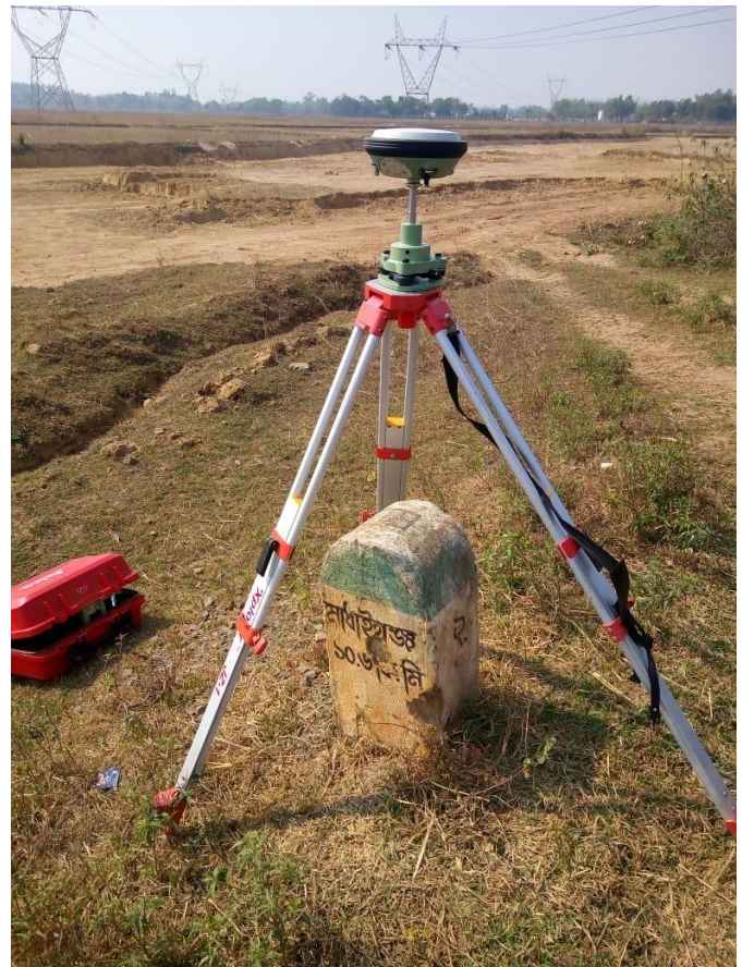
Plate 8: Subsidence monitoring station at ES19C
