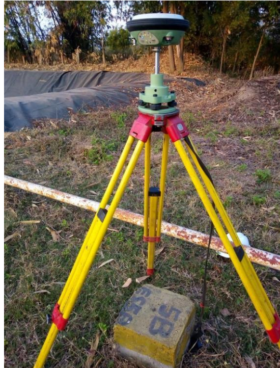
Plate 2: Subsidence monitoring station at ES5B
