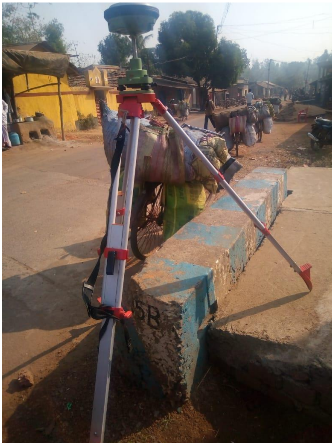
Plate 7: Subsidence monitoring station at ES15B
