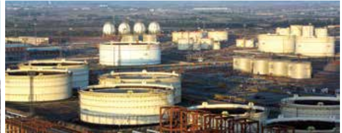
Tankages & Terminals Crude Oil, Intermediate, Finished Product
