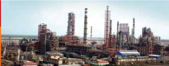
Hydrocarbon Refinery, Petrochemical, Fertilizer
