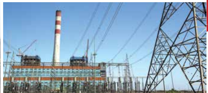
Power Plants Coal, Combined Cycle, Multi-fuel, Hydel
